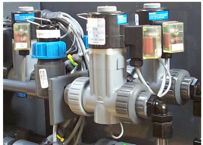
New Valves Installed In VUE 5
